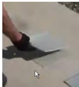
PLACING SECOND PAD
